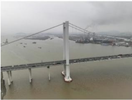
(a) Original bridge image
