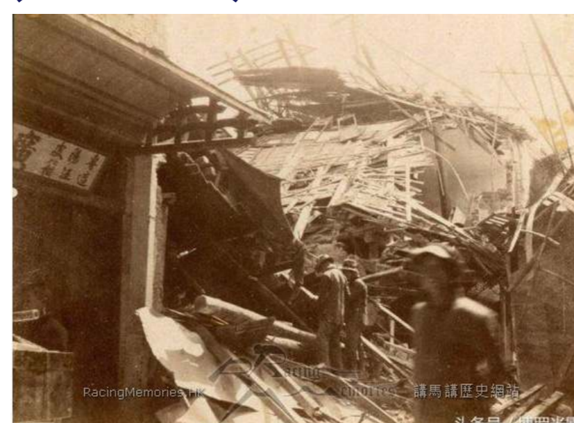
Damaged buildings during the 1918 Shantou Earthquake
