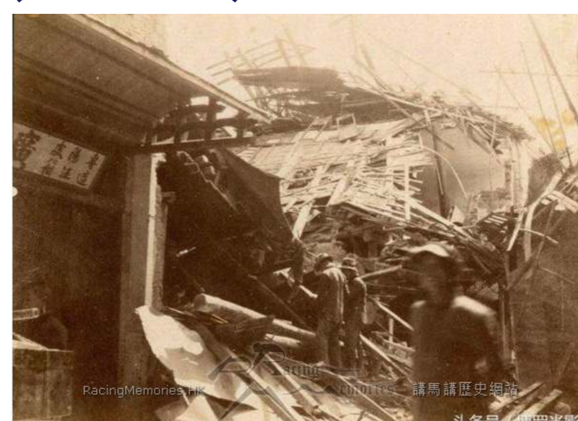
Damaged buildings during the 1918 Shantou Earthquake
