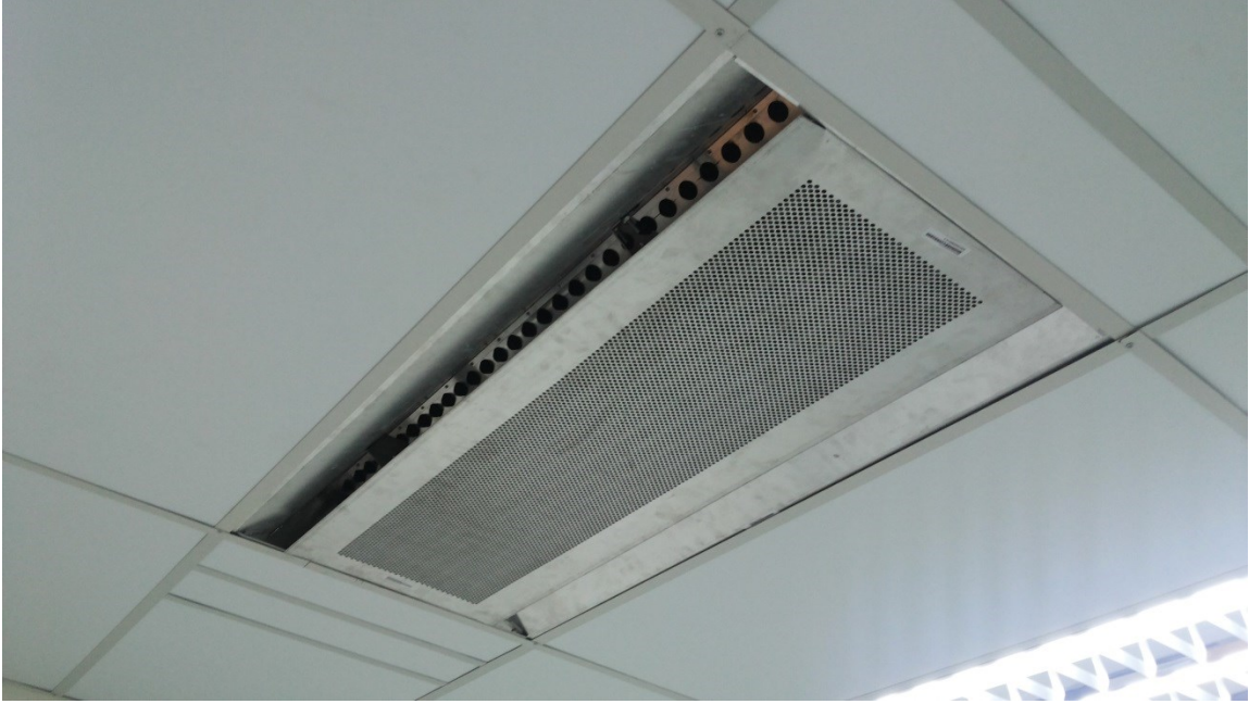
Photo of Active Air Terminals
