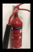
Carbon dioxide type fire extinguishers are used to put out Class B fires. Found only in certain SPMS laboratories
