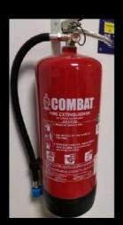
Water mist type of fire extinguishers are used to put out Class A, B & F fires. Found only in certain SPMS laboratories
