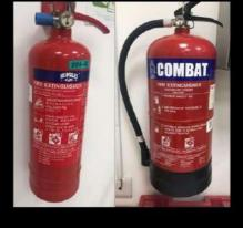
Dry powder type fire extinguishers are used to put out Class A & B fires. Widely available in SPMS offices and laboratories
