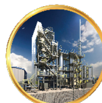
Residues and Resource Reclamation Centre
