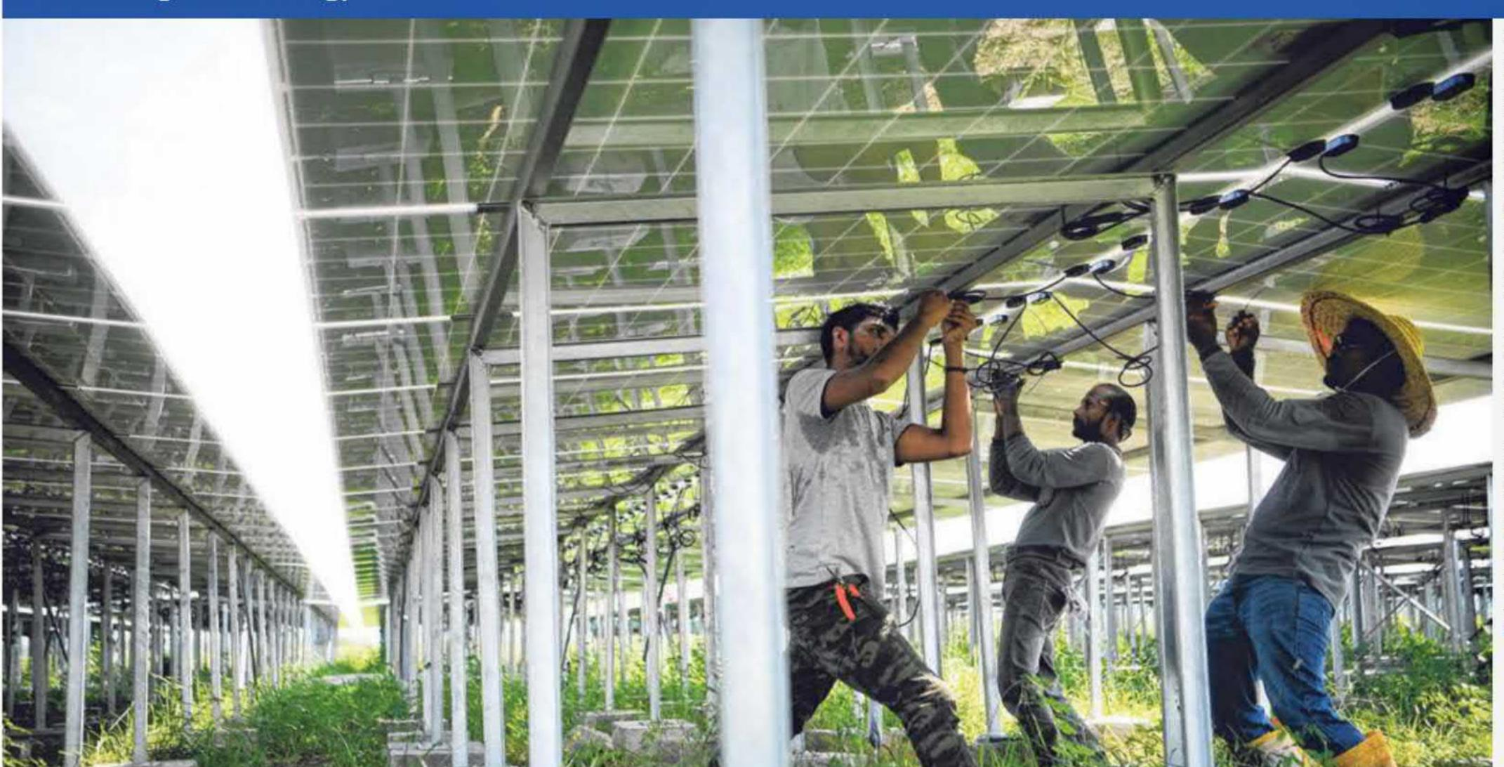
These rows and rows of solar panels, some of which are being adjusted by workers, on Semakau Island help to power a deep-sea fish farm there running on 100 per cent clean energy. They are part of the Renewable Energy Integration Demonstrator-Singapore (Reids), which integrates energy from micro-grids powered by light, the wind and even tides, and can be used to generate power in remote areas.
