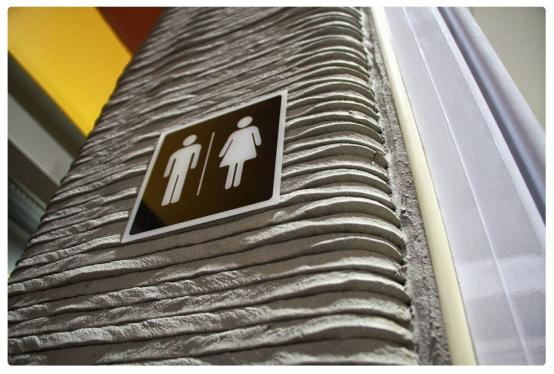
A closer look at the prefabricated bathroom unit's texture, which was formed by repeated layers of the W-lattice shape. — TODAY pic
