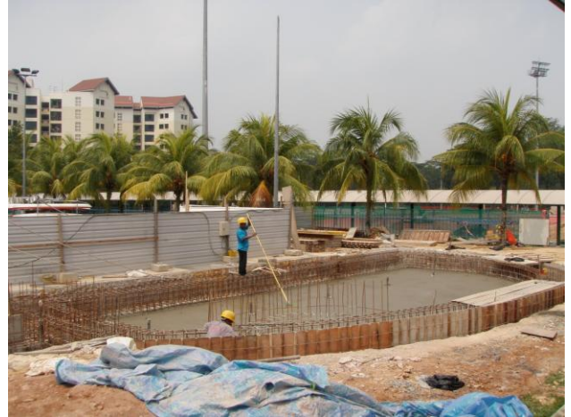
Construction works of the new wading pool
