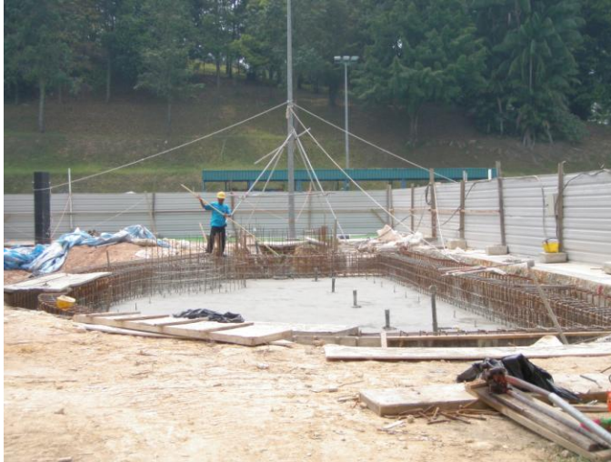
Construction works of the new wading pool
