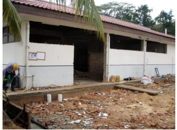
View of Swimming Pool Renovation
