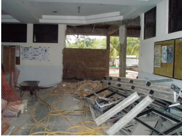
Hacking Works to the Swimming Pool Toilets
