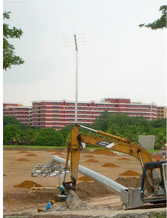
Erection of light mast & light fitting
